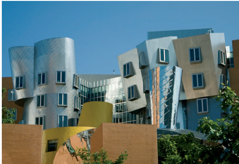
Ray e Maria Stata Center, Massachusetts Institute of Technology, Cambridge, USA
